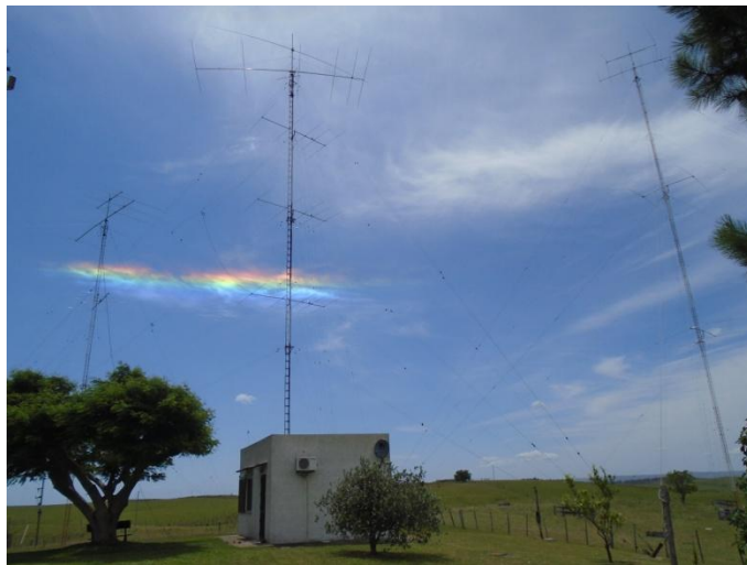
The impressive antenna arrays at CW5W. (Photo credit – Jorge, CX6VM)
